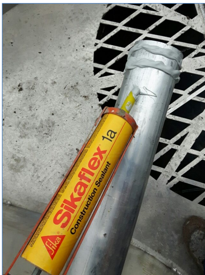
FIGURE 5 : GASKET ON OIL PIPE
